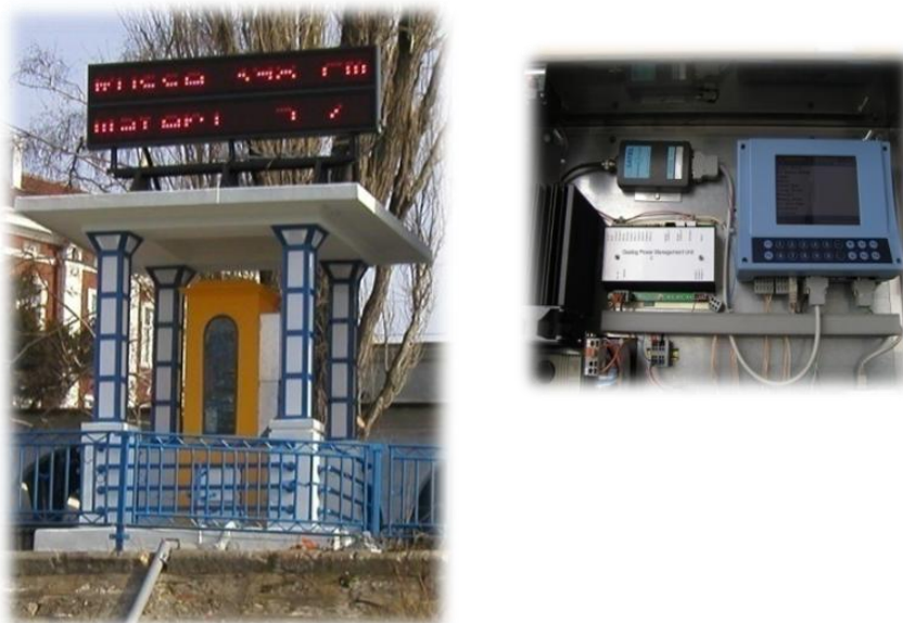
Figure 3 - Self-writing water measuring gauge in Ruse
