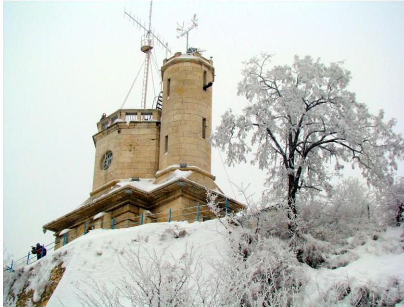
Figure 2 – Hydrometeorological station in Ruse
