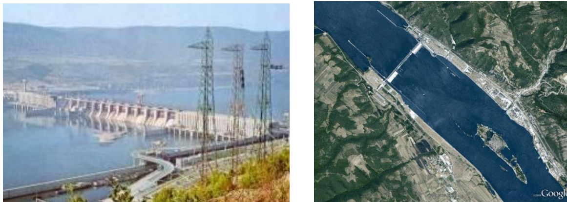
Figure 10. hydroelectric power station – km 943 /Iron Gate 1
