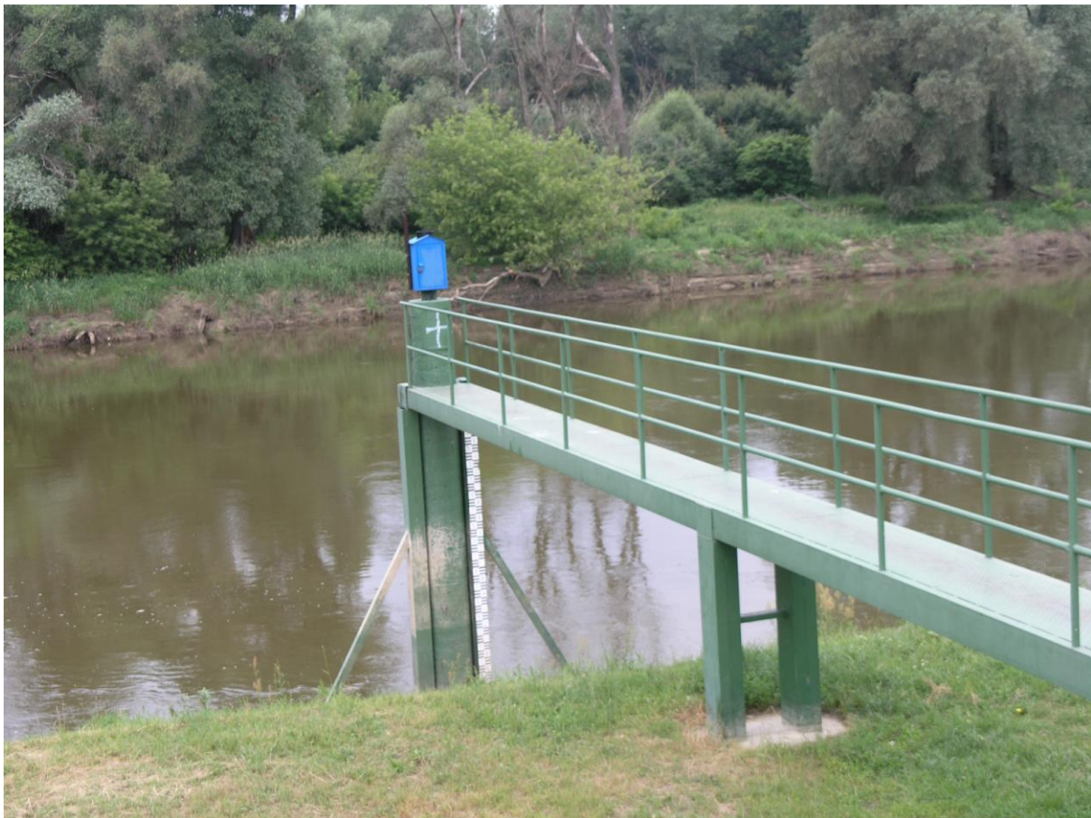
Fig. 2 Water gauge station
