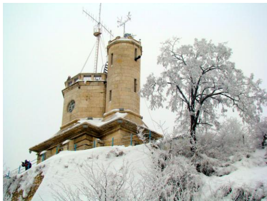
Figure 4 - Hydrometeorological station in Ruse
