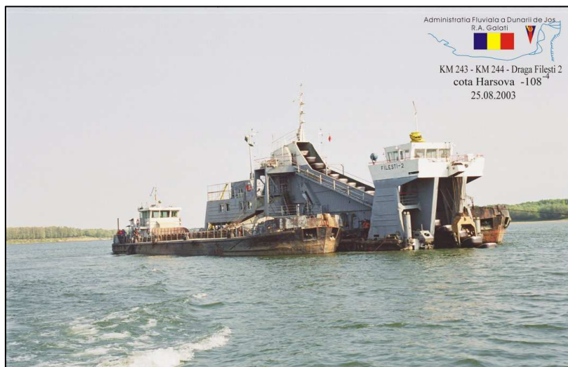
Bucket dredger 750 m 3
