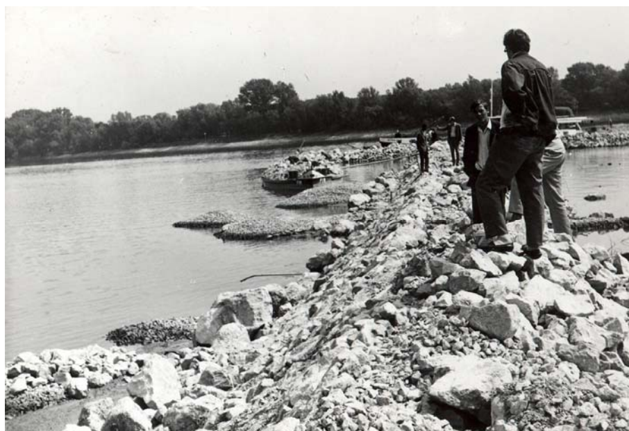
Photo 4: River training works performed during 1970s
